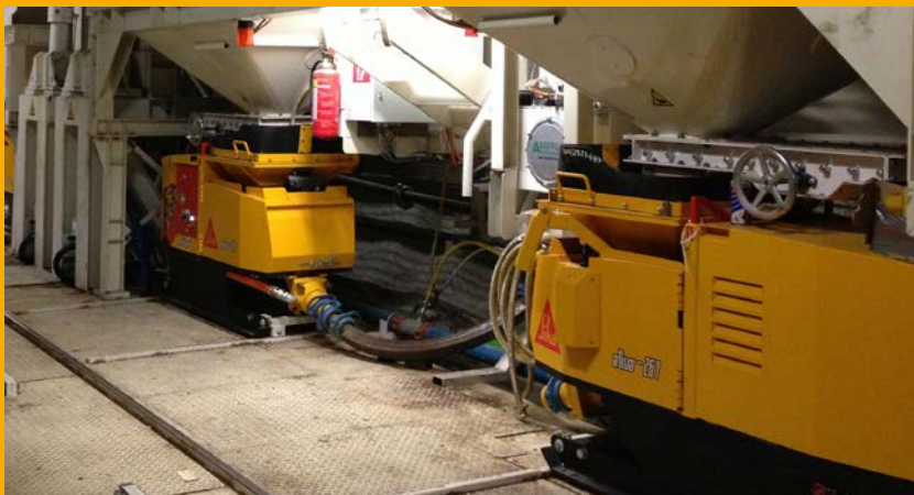
Pea gravel backfilling installation on TBM
