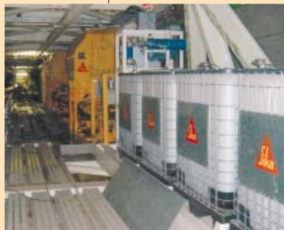
Concrete transfer station and admixture containers
